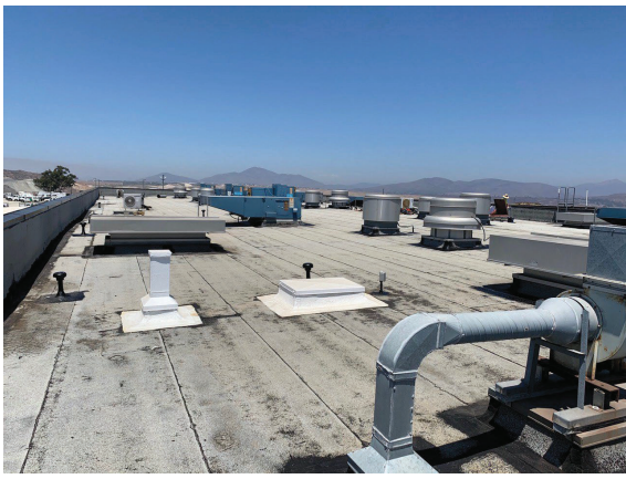
1. Cap Sheet roof cleaned for SRR System
