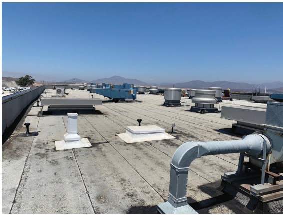
1. Cap Sheet roof cleaned for MREC System
