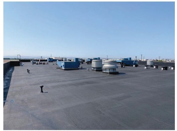
2. Cap Sheet coated with IPP Rubber
