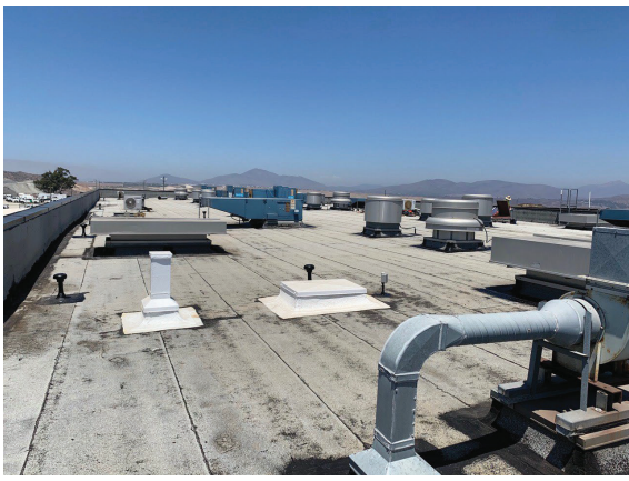
1. Cap Sheet roof cleaned for SRR System
