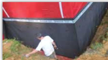
Installation of Waterproofing Plus System with water shield
