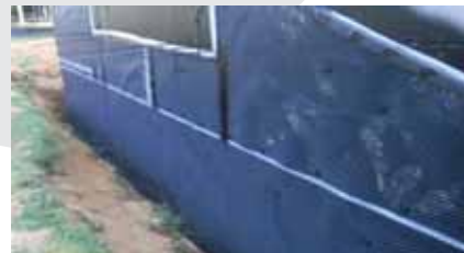
Installation of Waterproofing Plus System
